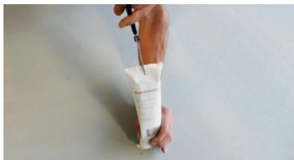
1 Cut a small hole at the top of the Skamol Glue bag.
