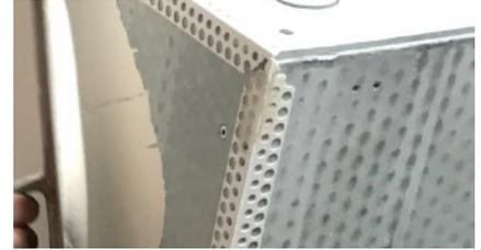
**3** Clip Skamol Corner into the plaster. Even out excess plaster.
