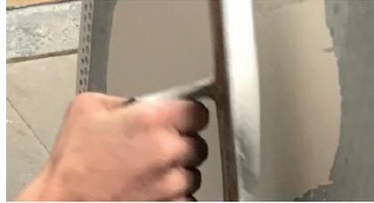
**2** Mix and apply Skamol Structural Plaster or Skamol Smooth Plaster, where Skamol Corner is placed.
