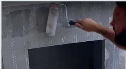
**2** Apply Skamol Primer on the surface of the SkamoEnclosure Board where the plaster is to be applied.
